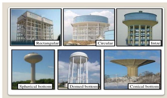
Fig. 1 Types of water tanks
