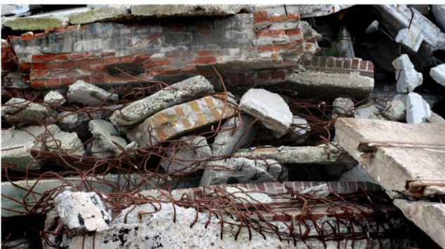
Figure 2: Old concrete and other building materials
